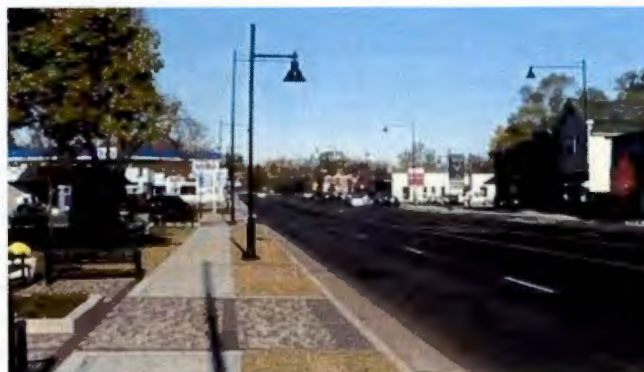
Figure 77. Example streetscape project in small town
