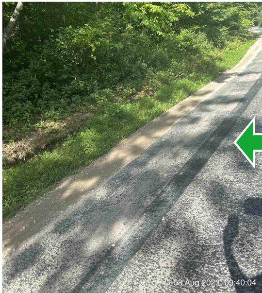
Beechland Rd / Jones Drive Shoulder Repairs
