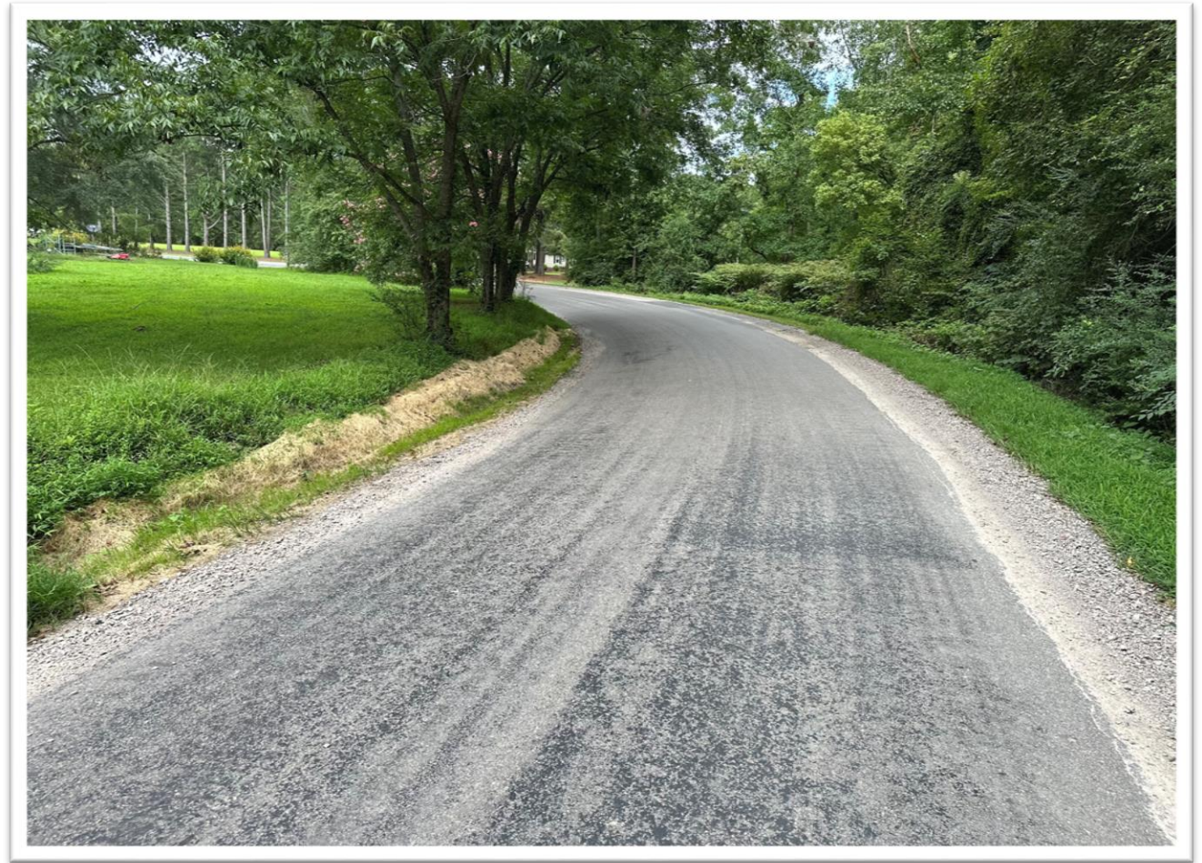
Ditch repair, seeding, and shoulder work along Bellevue Road
