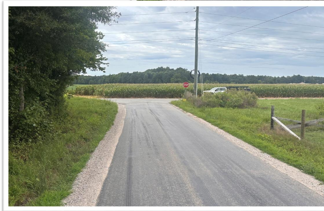
Additional shoulder repair on Bellevue Rd
